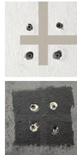
**5** Mask the grounding plate, it is not allowed to overpaint it! **Overpaint the area with commercial wall paints**, wallpapers or use fine plaster as recommended in the corresponding technical data sheets.
